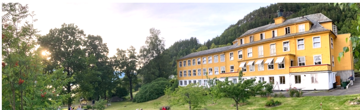
Jonatunet, built in 1934 as a tuberculosis nursing home. From health for the body, to health for the mind as a psychiatric institution, today health for the globe: Nordic center for peace, development and the environment.
